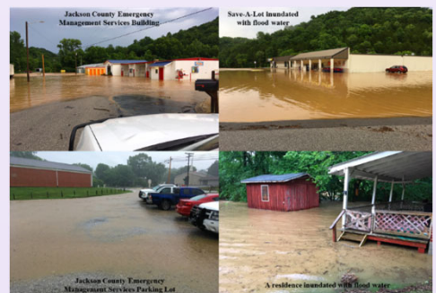
Figure 1. June 27, 2018 Flooding in Jackson County (Source: Town of Gainesboro)
