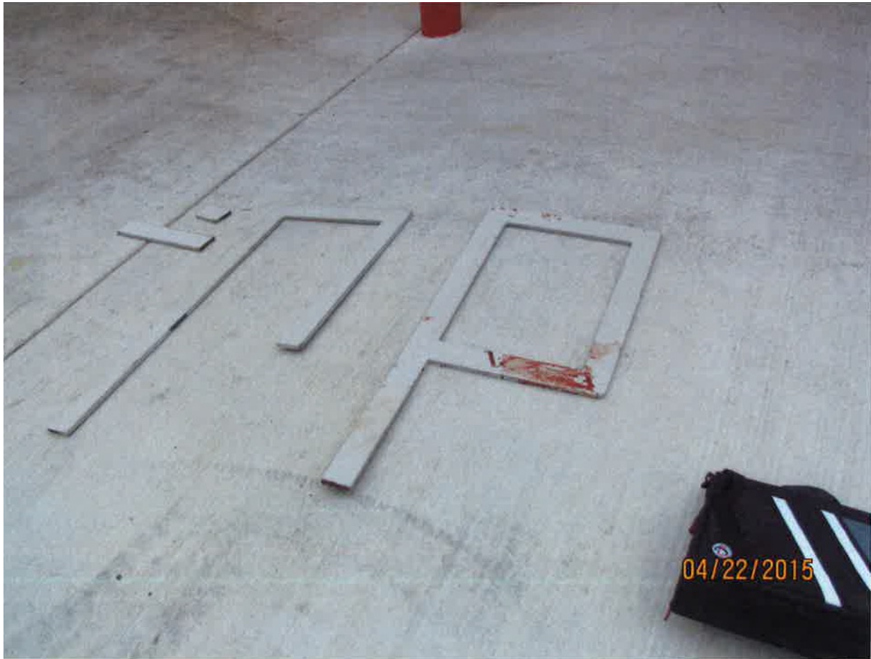
Photo 2 of 2 – This photo shows the upper grab rails of the ladder that broke free from the fixed building ladder.
