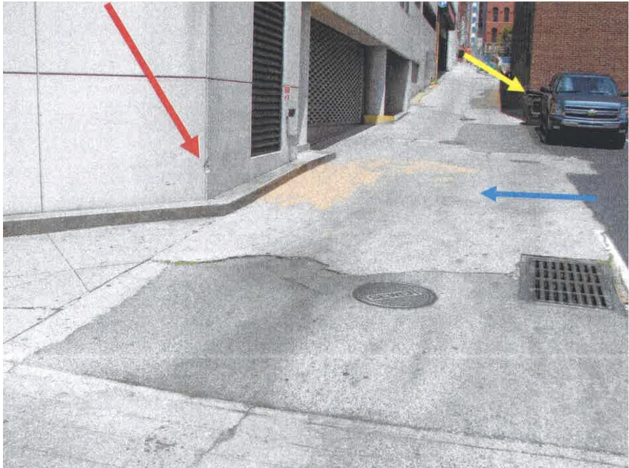
Photo 2 of 2 – The red arrow shows the location of impact with the rear passenger side of the truck and the building. The yellow arrow shows the location of trash cans that were being collected. The blue arrow shows the approximate location where the truck stopped.
