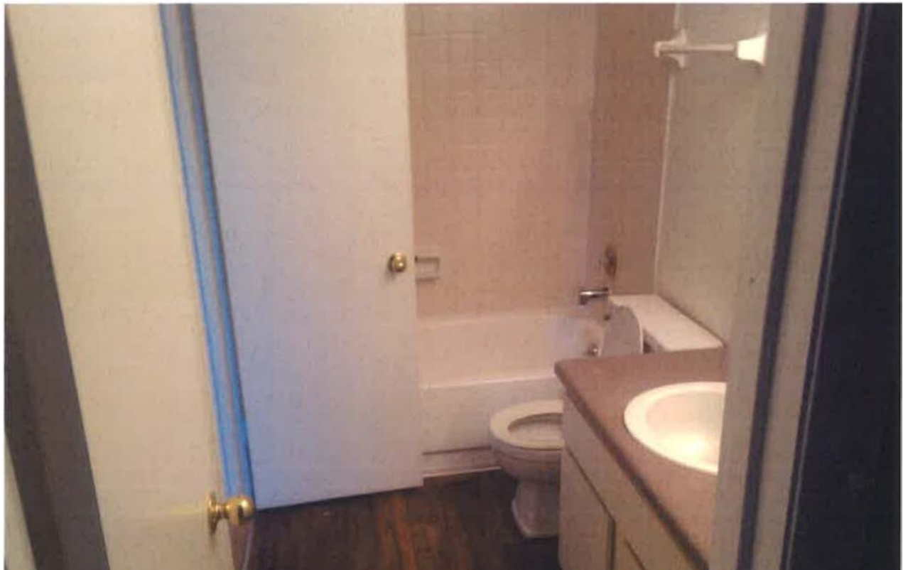
Photo 1 of 1: View of the bathroom where employee was re-finishing the bathtub using a chemical stripper containing methylene chloride. The victim was found inside the bathroom with both the laundry room and hallway doors closed.
