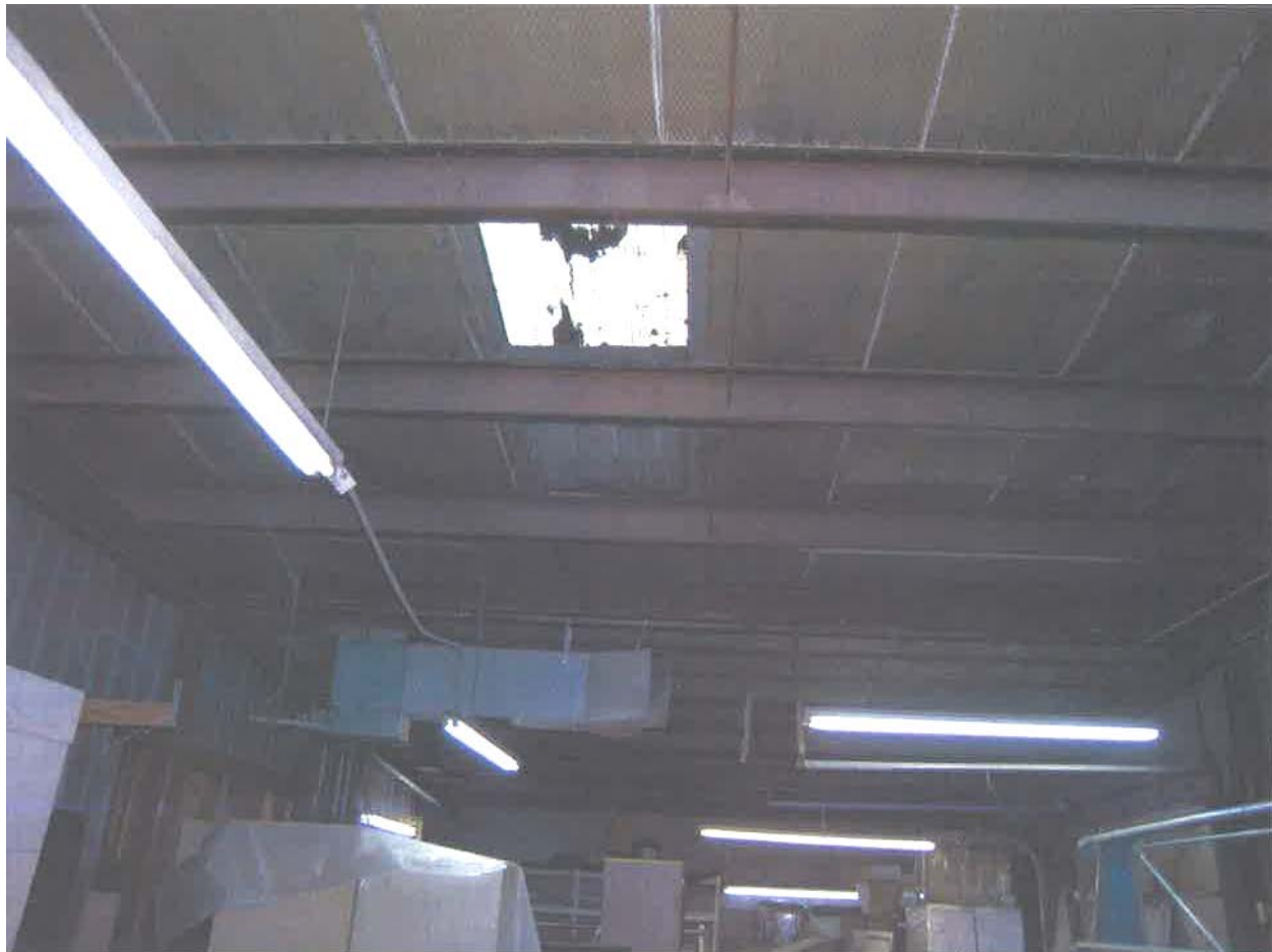
Photo 1 of 1 – Fiberglass skylight panel and the roofing tin cover.
